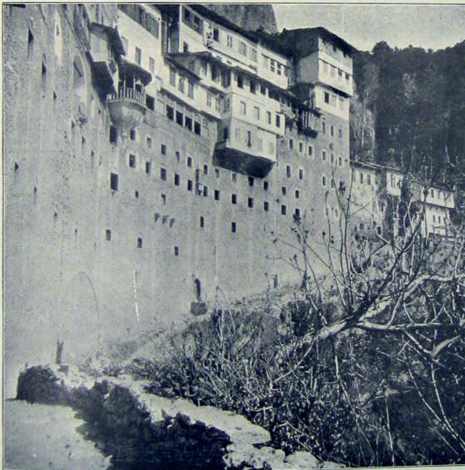
THE CELLAR WALLS
